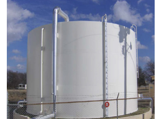
Water Storage Facilities
