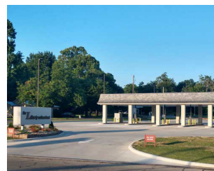
Commercial / Industrial Development
