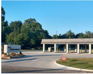
Commercial / Industrial Development
