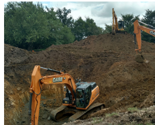
Surveying Services - Construction Layout
