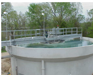
Water Treatment Plants
