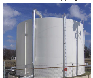
Water Storage Facilities
