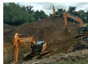
Surveying Services - Construction Layout
