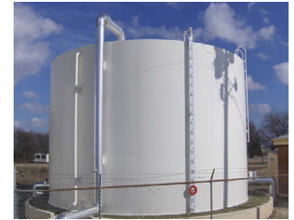
Water Storage Facilities
