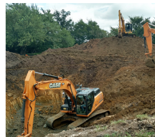
Surveying Services Construction Layout
