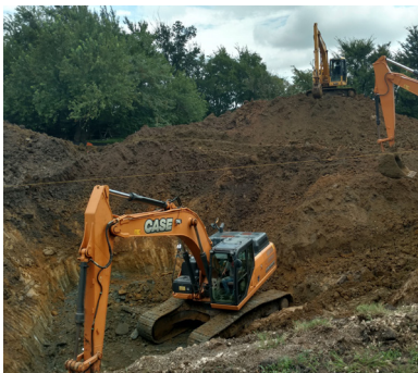
Surveying Services - Construction Layout
